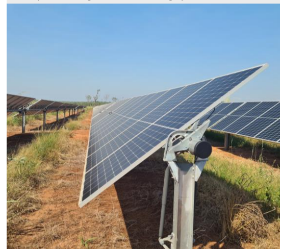
Example of a single axis tracking system
