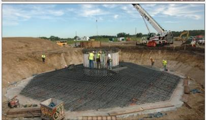
Tower foundations: ~800m³ concrete.
