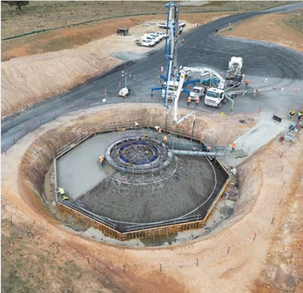
Foundation pour: Rye Park Wind Farm Source: Zenviron
