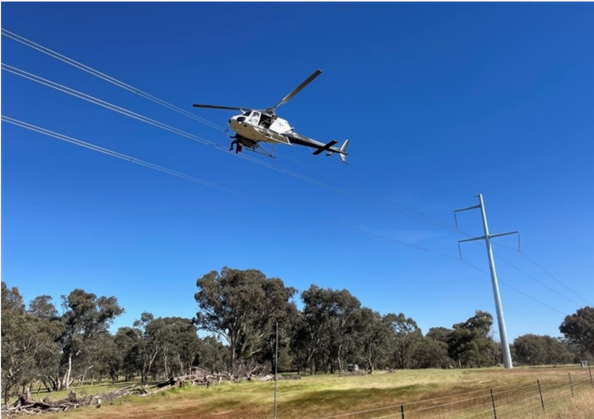
Helicopter Stringing powerline: Rye Park Wind Farm Source: Zenviron
