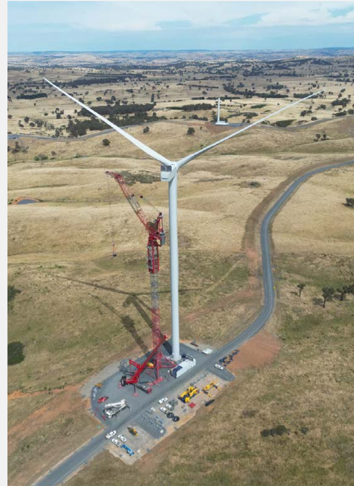
Tower crane: Rye Park Wind Farm Source: Zenviron
