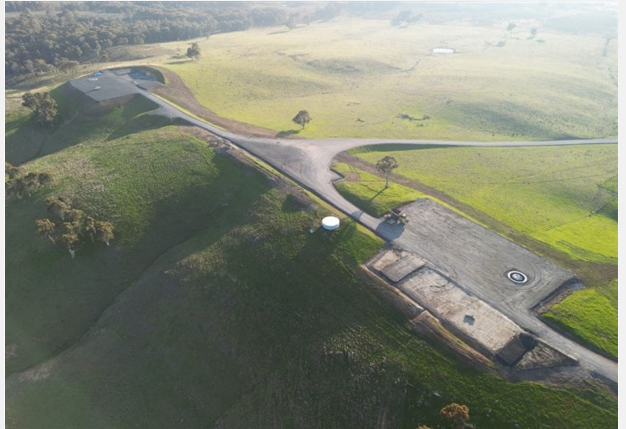
Completed hardstand: Rye Park Wind Farm Source: Zenviron
